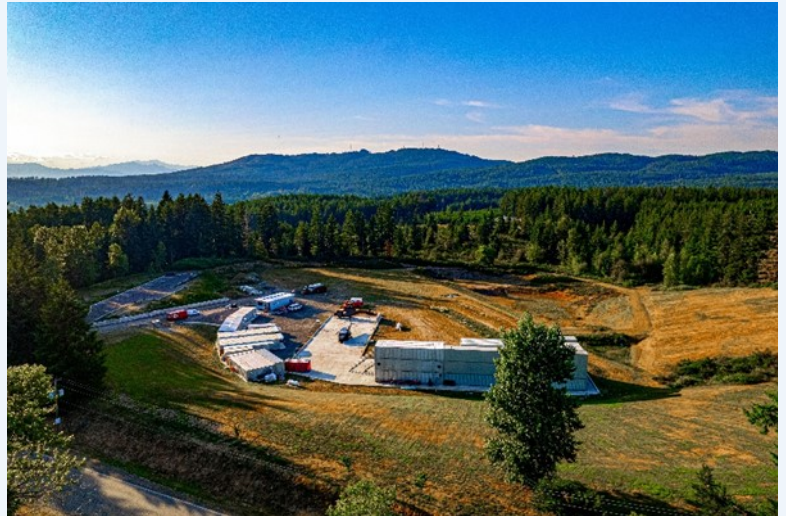
Bremerton Marina (top) and Olympic View Industrial Park (bottom)
